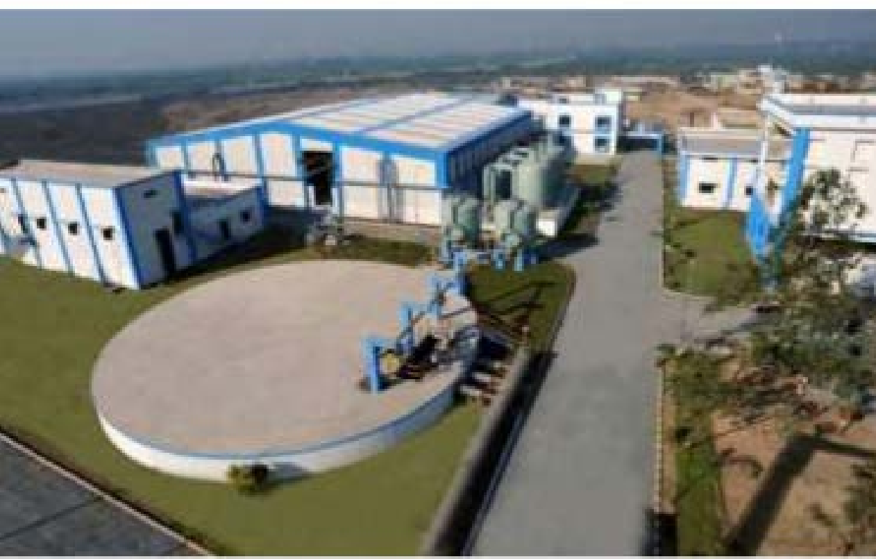
Bamroli Tertiary Treatment Plant
