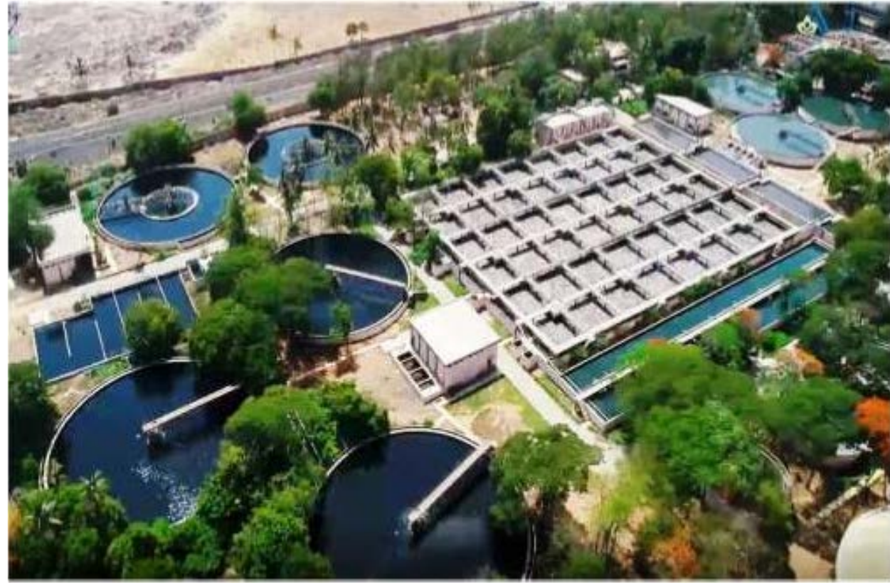
Anjana Sewage Treatment Plant
