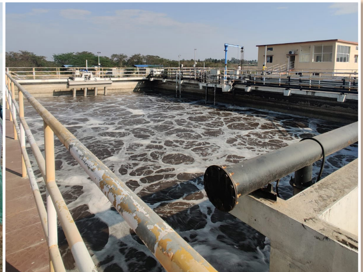
MoHUA team led by Dr. VK Chaurasia, Joint Adviser, PHEE, CPHEEO visited the STP at Tirumalakudu in Narsipura, Mysuru district. The plant was established in 2019 with a capacity of 5.5 MLD using MBR technology. Catering to over 35,000 population, the plants treats around 3.6 MLD of sewage.
